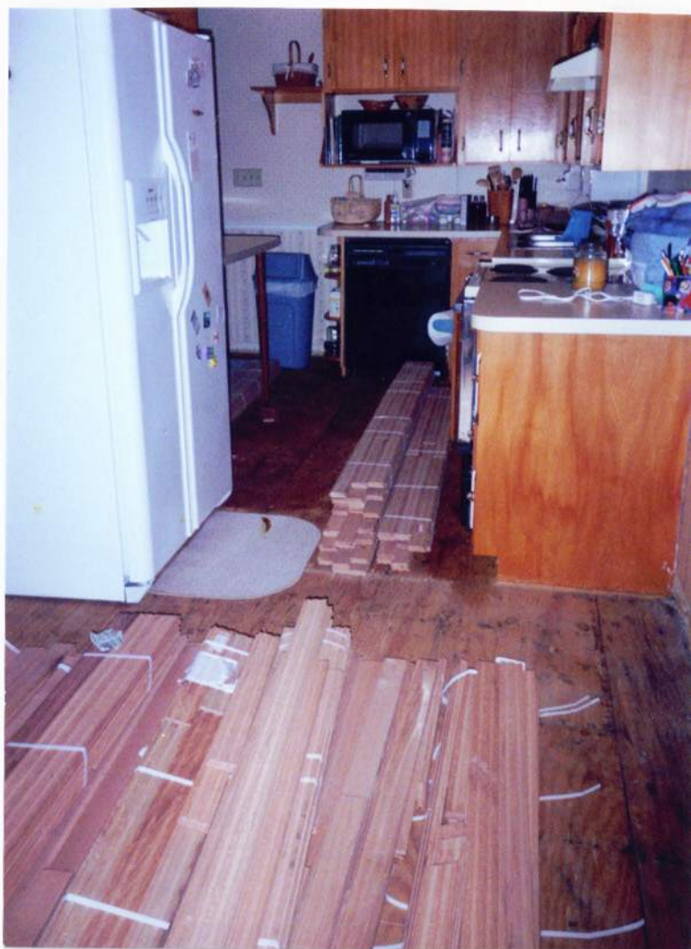
The Wilson house during May
